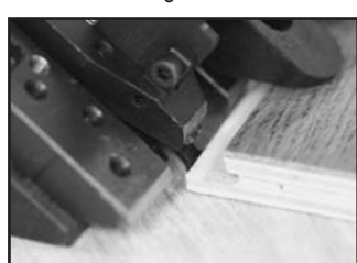
Fig. 15 Pin placed outside locking element - incorrect
